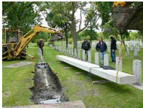
Figure 5. Installation of reinforced concrete beam on piles
