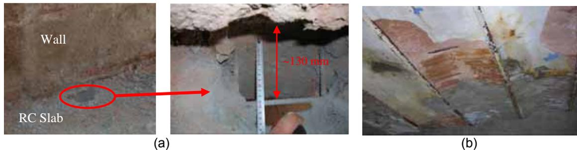
Figure 4. a) The connection of existing walls and reinforced concrete slabs of Block B, b) original vaulted slabs in Block E.
