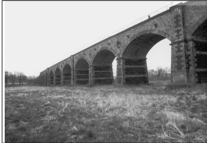
Railway viaduct Zittau, Germany
