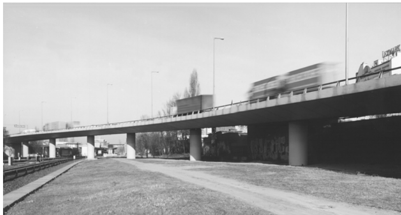
Westend bridge Berlin, Germany
