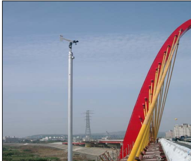
Wind Sensor at Taichung Bridge, Taiwan
