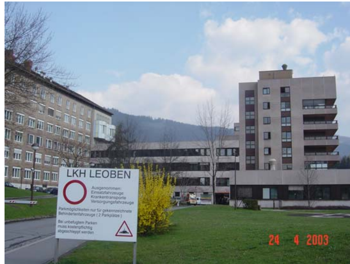
Hospital Leoben, Styria, Austria
