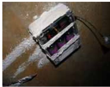
(b) Sensor Installment under Bridge
