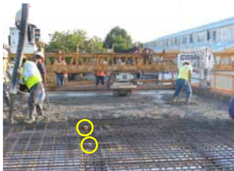
Figure 1. Prototype sensors attached to reinforcement in bridge deck.
