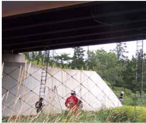
Figure 1. Crew setting up to measure cracks in bridge deck.
