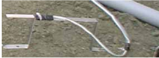
Figure 4. b) A Sensor Before Placing Concrete
