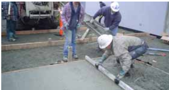
Figure 3. (a) Concrete Placement and (b) Finishing [Notice the sensors in (a)]
