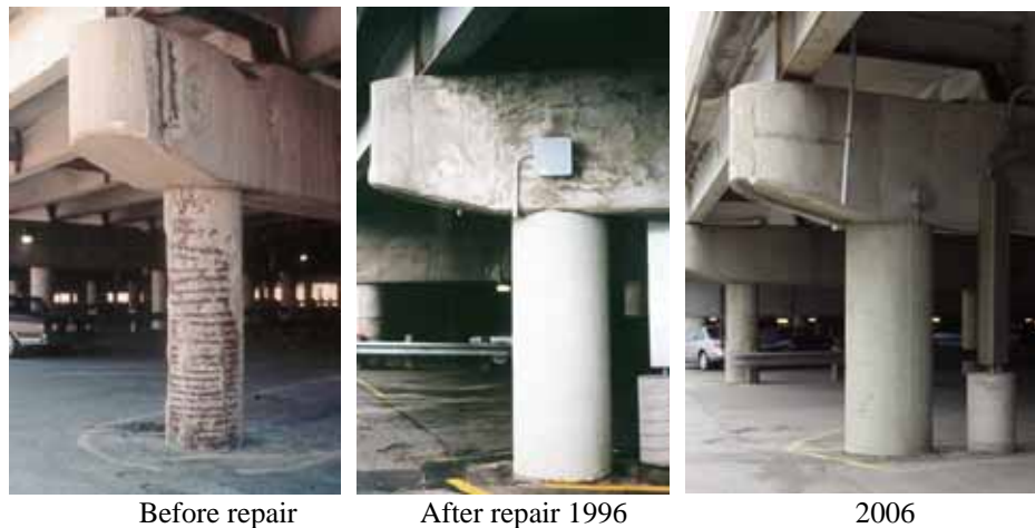
Figure 5. Columns before and after repair.
