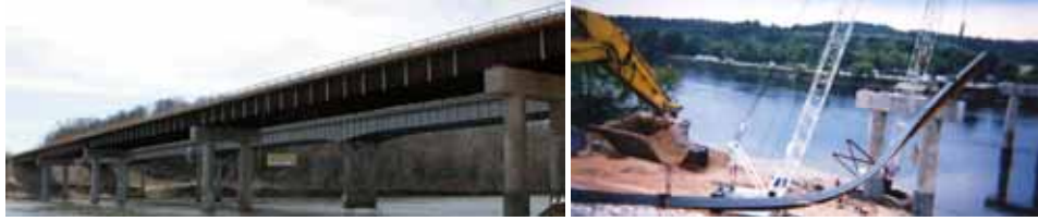
(a) Five-span continuous bridge
