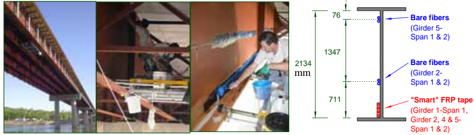
(c) Installation of a “smart” tape and two bare fibers
