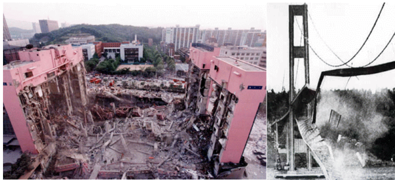
(a) Sampoong Department Store (1995, Korea) (b) Tacoma Bridge (1940, USA)
