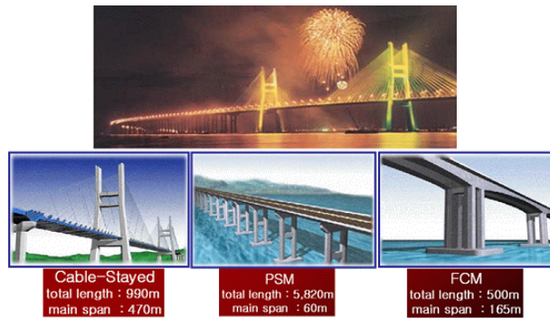
Figure 5. Bridge Type by Section, Seohae Grand Bridge (Korea)
