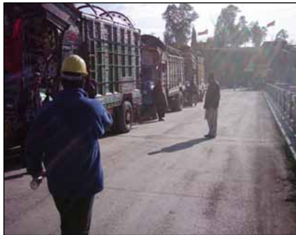
Figure 7: Three trucks loaded on the bridge
