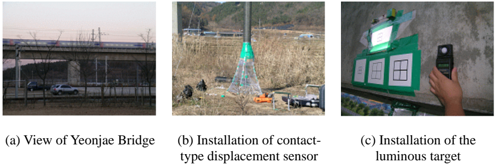
Figure 10. Contact-type and non-contact-type displacement measurement systems installed in Yeonjae Bridge
