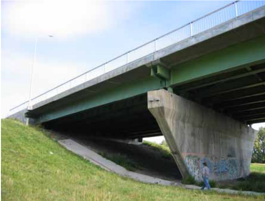
Picture1 Steel Free Deck Span in the North Perimeter Highway Red River Bridge
