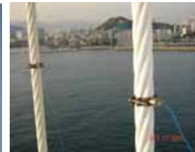
Figure 7. Accelerometers attached on hanger cables
