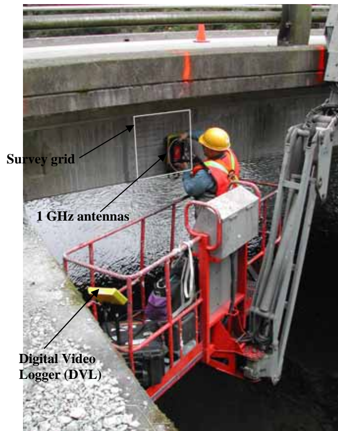
Figure 1. GPR scanning of a bridge girder.
