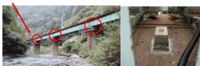
Figure 2.: Clinometric type scour monitoring device
