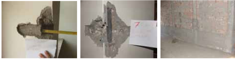
Figure 9. Field verification of design data.
