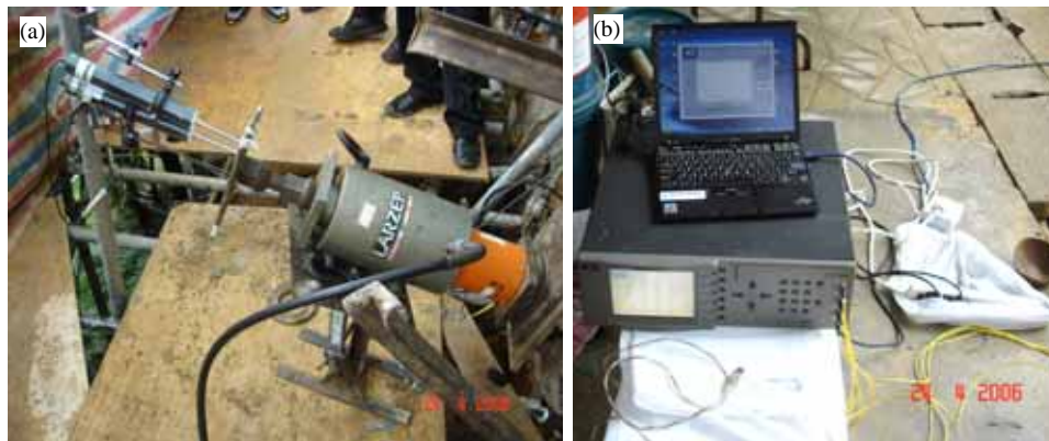
Figure 6. Soil nail pull-out test in Lantau Island of Hong Kong – (a) the pull-out setup and (b) the Micron Optics SI 425 Swept Laser Interrogator
