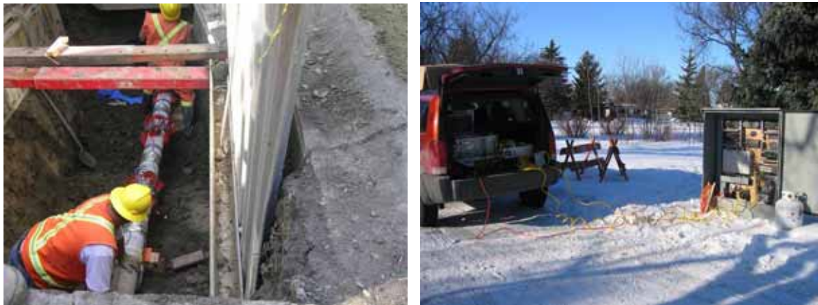
Figure 1. Installation of Instrumented AC Pipe Section Figure 2: Data Acquisition System.
