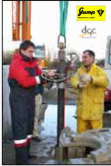
Figure 2. Installing the anchor.
