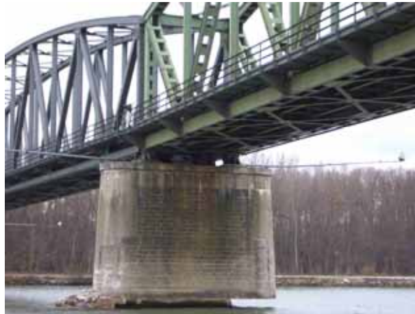
Figure 1. Damaged pier
