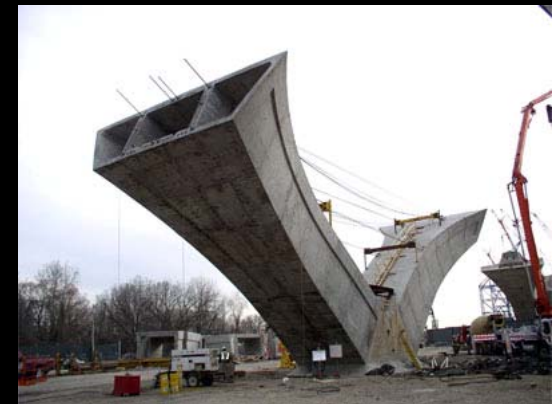
Woodrow Wilson Bridge Maryland-Virginia Over the Potomac, 2007
