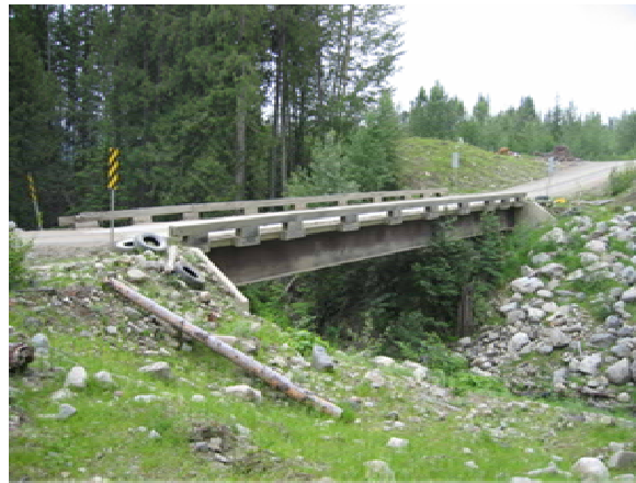
Figure 4a. Overview of the Lindquist Bridge.
