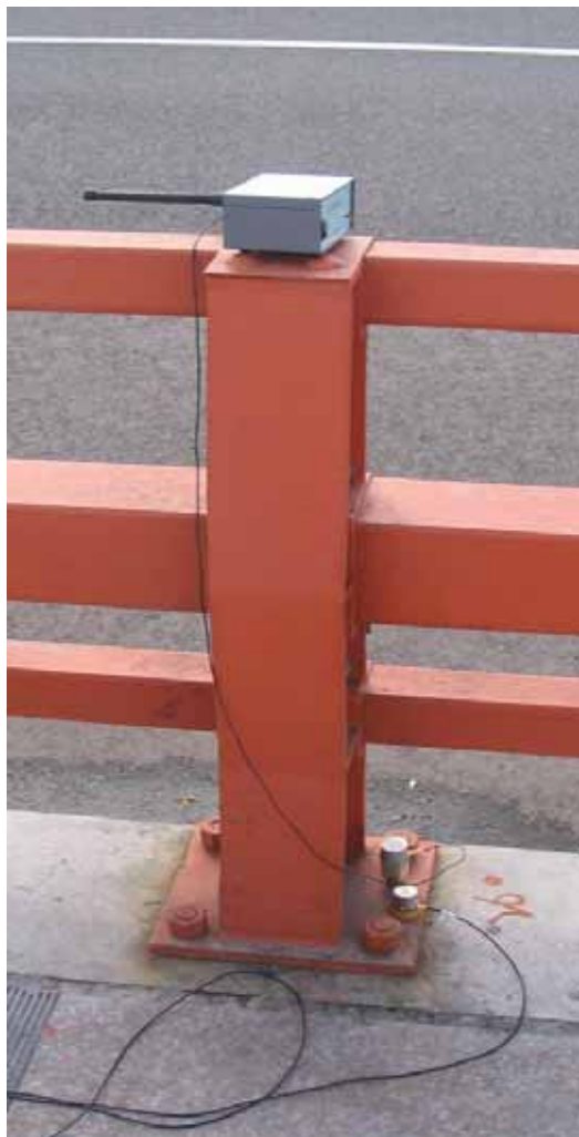
Figure 7 Wireless and cable-based accelerometers mounted on deck.
