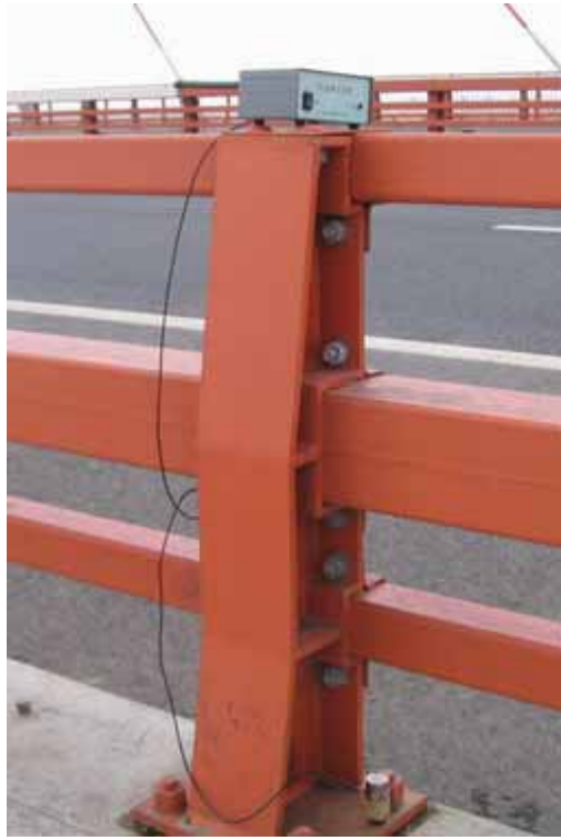
Figure 6 Vertical wireless accelerometers mounted on deck.
