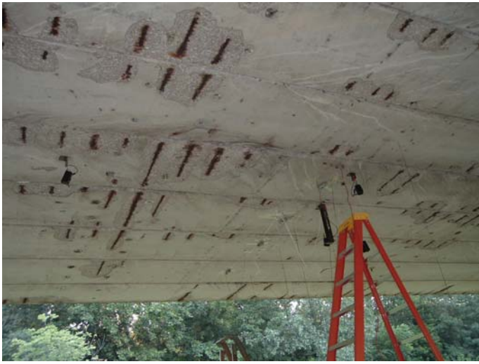
Figure 5. Photograph of the underside of the bridge span
