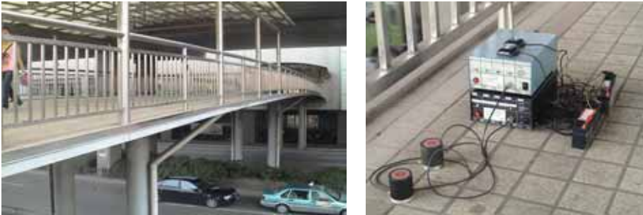
Figure 7 Vibration test of a steel structure footbridge
