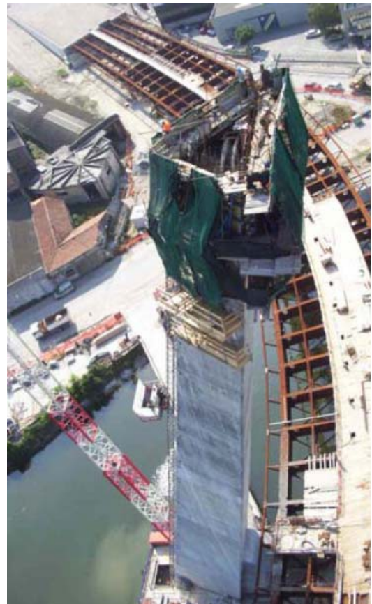
Figure 5 – View of the pylon during construction
