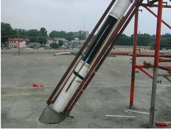
Figure 8 – Attachment of a SOFO sensor on the stay cable
