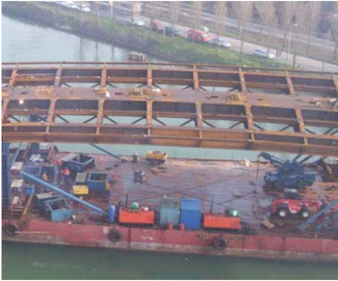
Figure 2 – View of the steel deck during transport
