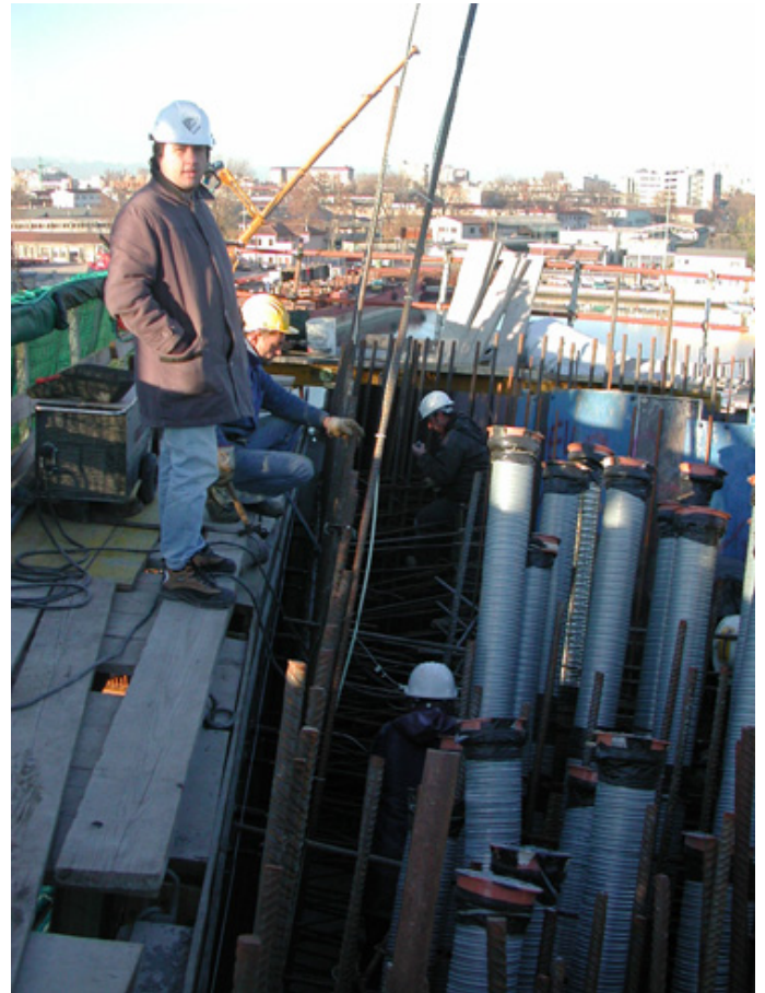
Figure 6 – Positioning of a SOFO sensor inside the pylon
