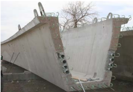
Figure 2. U-Shaped Bridge Girder with Eight Empty Ducts
