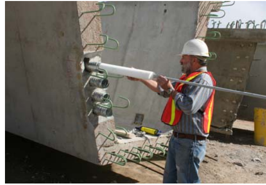
Figure 3 – Styrofoam rods being inserted into the duct
