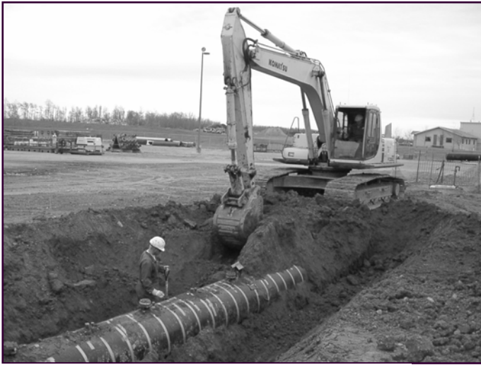
Figure 2. The excavation of the buried pipeline
