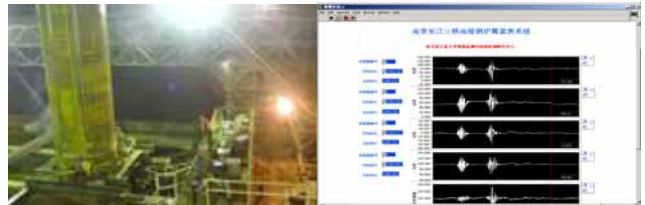
Figure 27. Construction monitoring for steel protective tube
