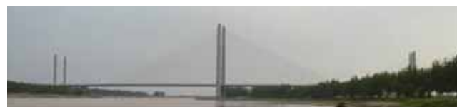
Figure 22. Binzhou Yellow River Bridge under monitoring
