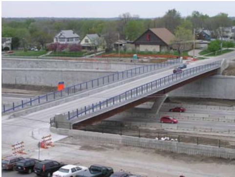
Figure 1. East 12 th Street Bridge as seen from the SHM site camera
