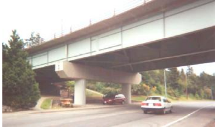
Figure 5. Portage Creek Bridge in Victoria, British Columbia
