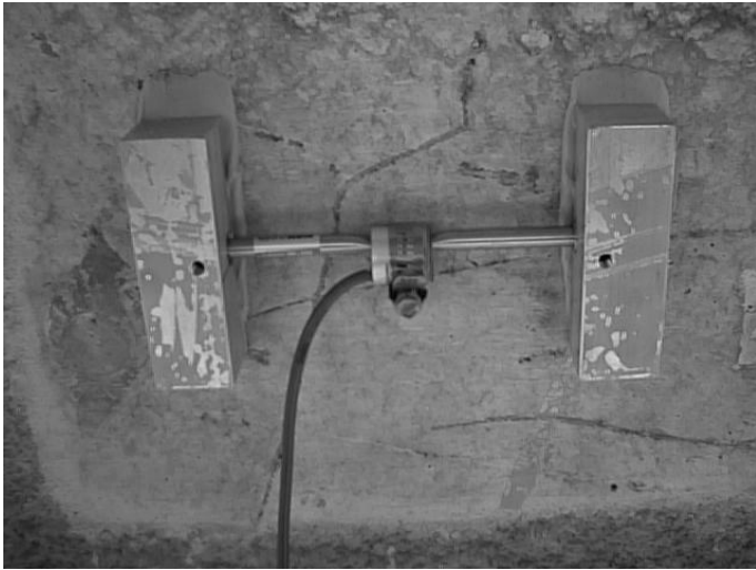
Fig 9 VW SG mounted onto surface of bridge
