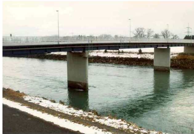
Bridge Oberriet - Meiningen, between Switzerland and Austria
