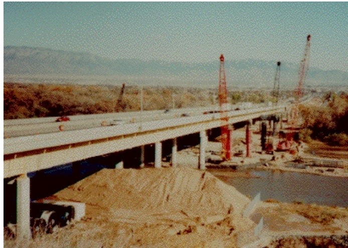
I40-Bridge, New Mexico, USA
