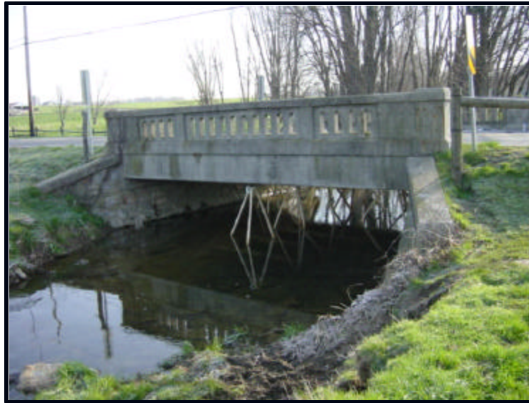
Figure 2: Representative reinforced concrete T-beam bridge
