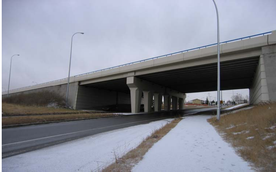
Figure 1: Beddington Trail Bridge - Calgary, Alberta, Canada
