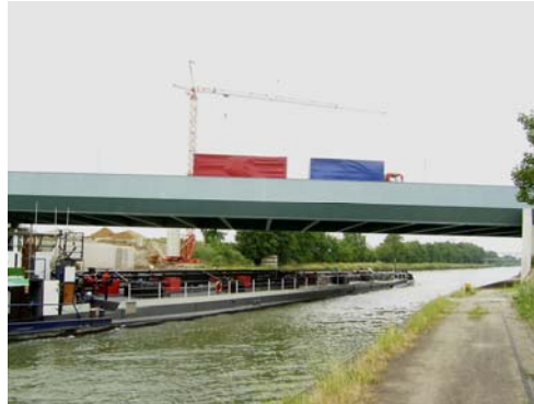
BW91 near Braunschweig, Germany
