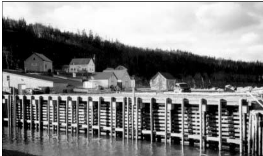
Figure 6.22 Hall's Harbour Wharf – Nova Scotia
