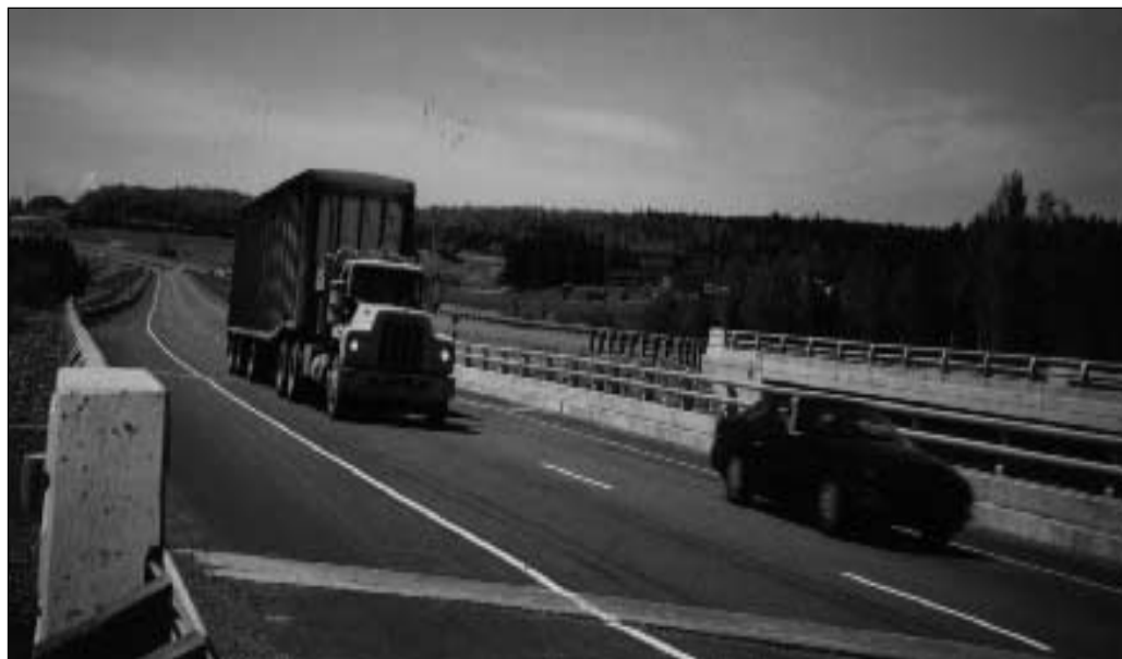
Figure 6.2 Salmon River Bridge – Nova Scotia
