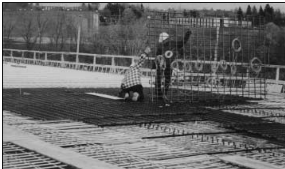
Figure 6.17 Joffre Bridge - Sherbrooke, Québec
