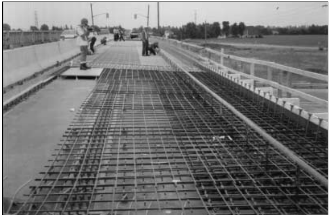
Figure 6.6 Installed sensors in steel-free deck with carbon fibre NEFMAC
