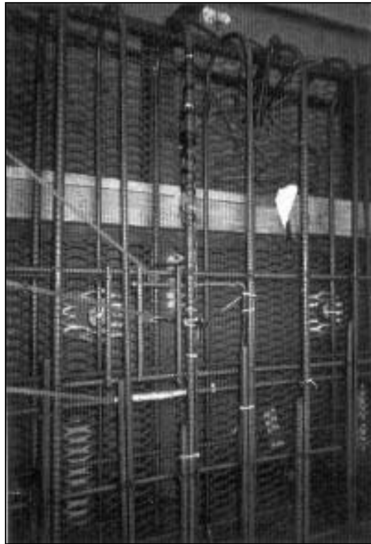
Figure 6.8 Photograph showing sensors installed on a rebar cage
